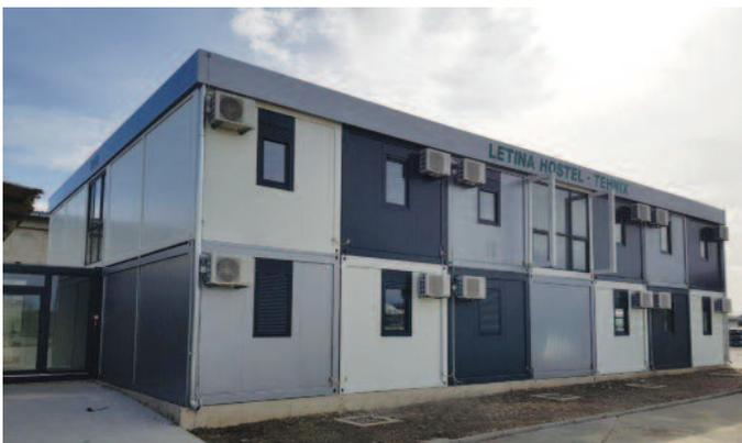
Modular Tehnix hostel with 100 accommodation units and built-in sanitary unit, kitchen and 4 beds
